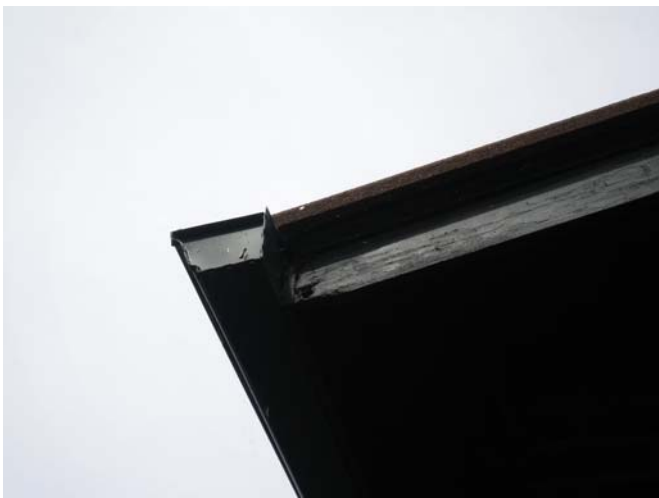
Rot at wood fascia
