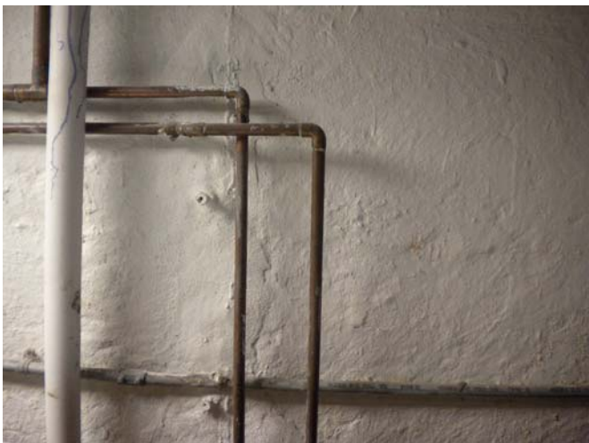
Epoxy grouted foundation crack
