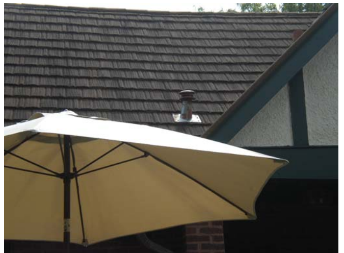
Flashing improper
